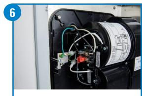
Connect electrical service to Terminal Block of hand dryer. Properly ground the dryer via the supplied ground screw.
