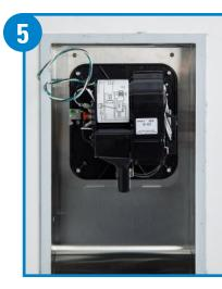
Knock out the appropriate electrical inlet on dryer wall plate and install dryer insides onto dryer mounting plate using all 6 mounting nuts supplied.
