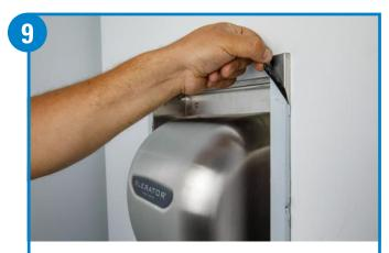
Return dryer to upright position and refasten to Wall Box using the 2 button head tamper proof bolts. Remove protective film from Wall Box. Turn on power and test for proper operation.
